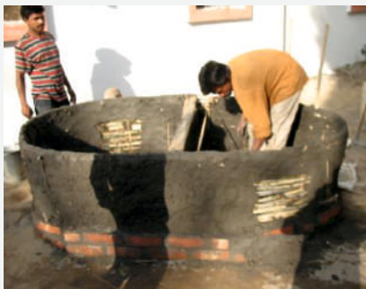
EcoSan toilet constructed using bamboo for flood affected areas
