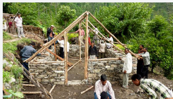
On-site discussions with construction workers during the training sessions.
