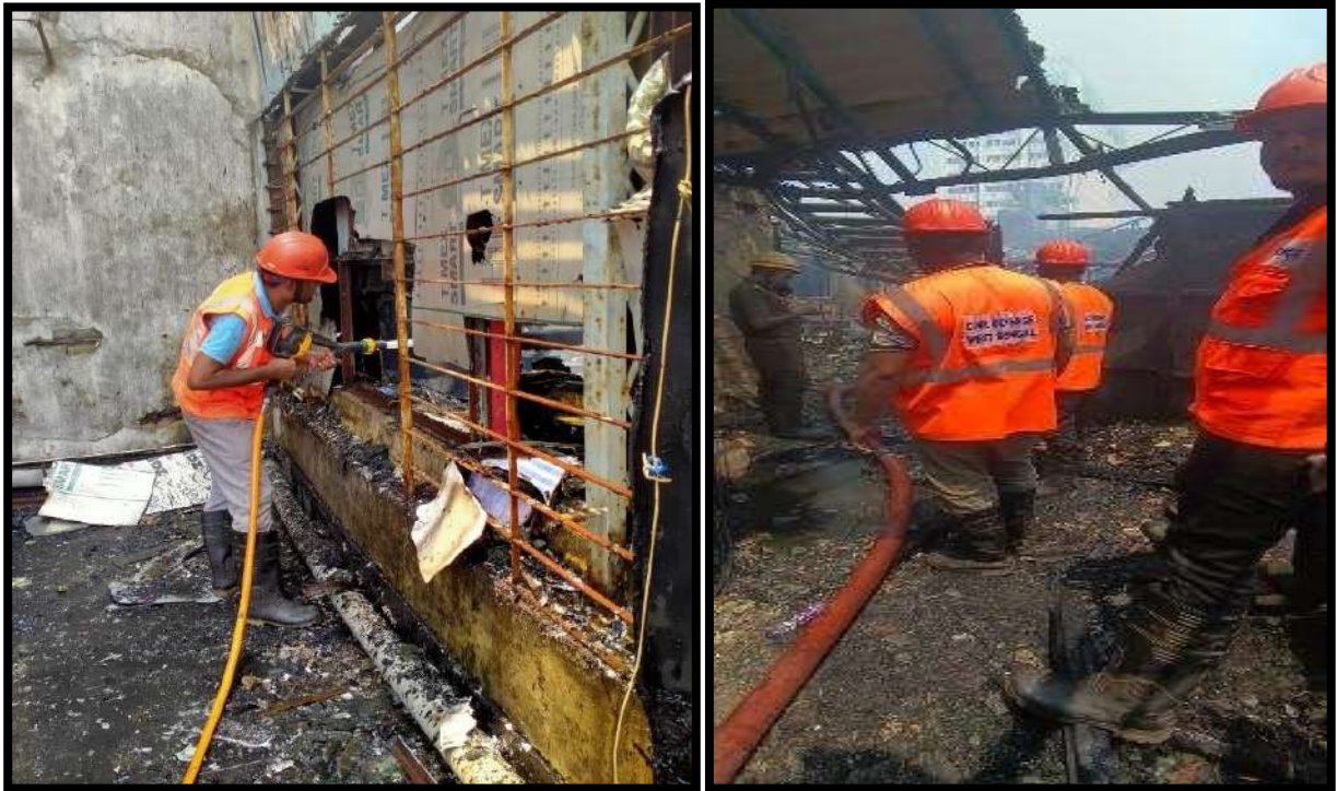
Fire incident at 4/1 Red Cross Place, 3rd floor Central Bank building Kolkata –70001
