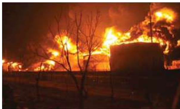
IOC Jaipur Depot during burn out, Jaipur
