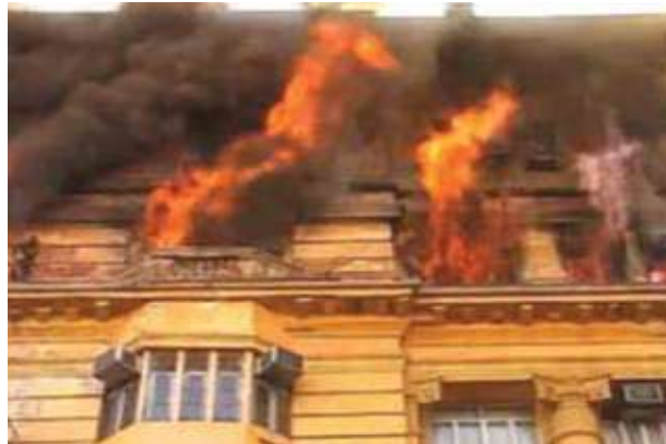
Park Street heritage building on fire, Kolkata
