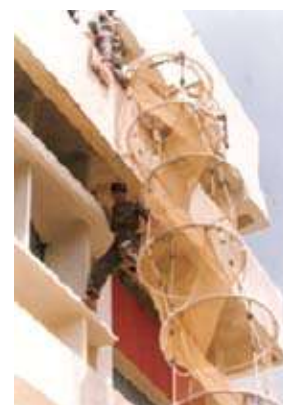
Emergency Escape Chute
