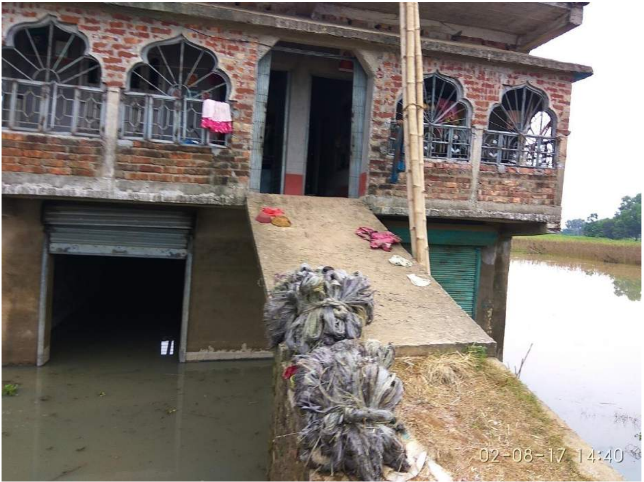
Figure 3: People evacuated ground floor and started shifting to 1st floor at Chabbisipur village, Khanakul 1 block, Hoogly.
