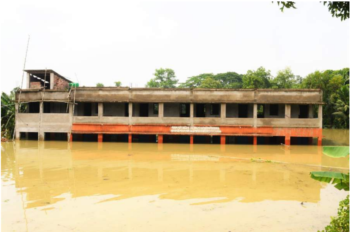
Figure 32 Village: Palashpai, GP: Kheput, Block: Daspur - II, Dist: PaschimMedinipur
