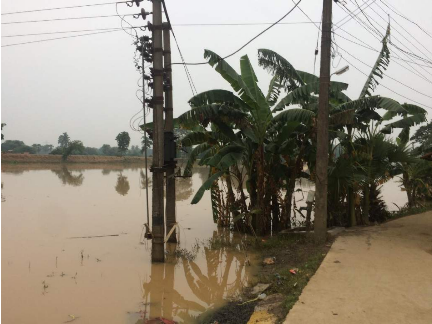
Figure 11 Electric Supply Faced Challenge at Village - Chitkola, Jangipara Block, District – Hooghly
