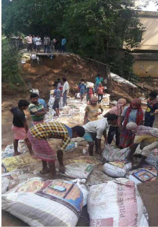
Repairing of Roads in Hooghly
