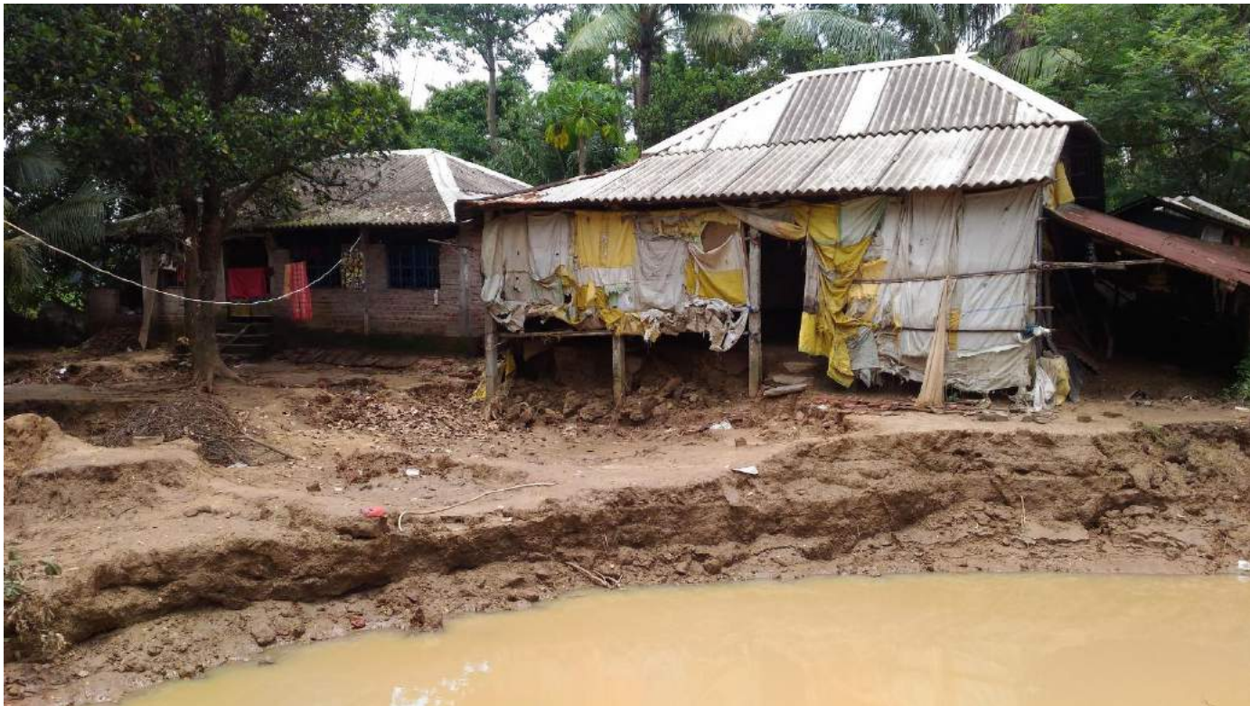
Figure 17 During Flood (25.07.17) River Damodar made it's path this way at atUttarnityanandapurSamitimana, Radhamohanpur GP, Block - Sonamukhi, Bankura
