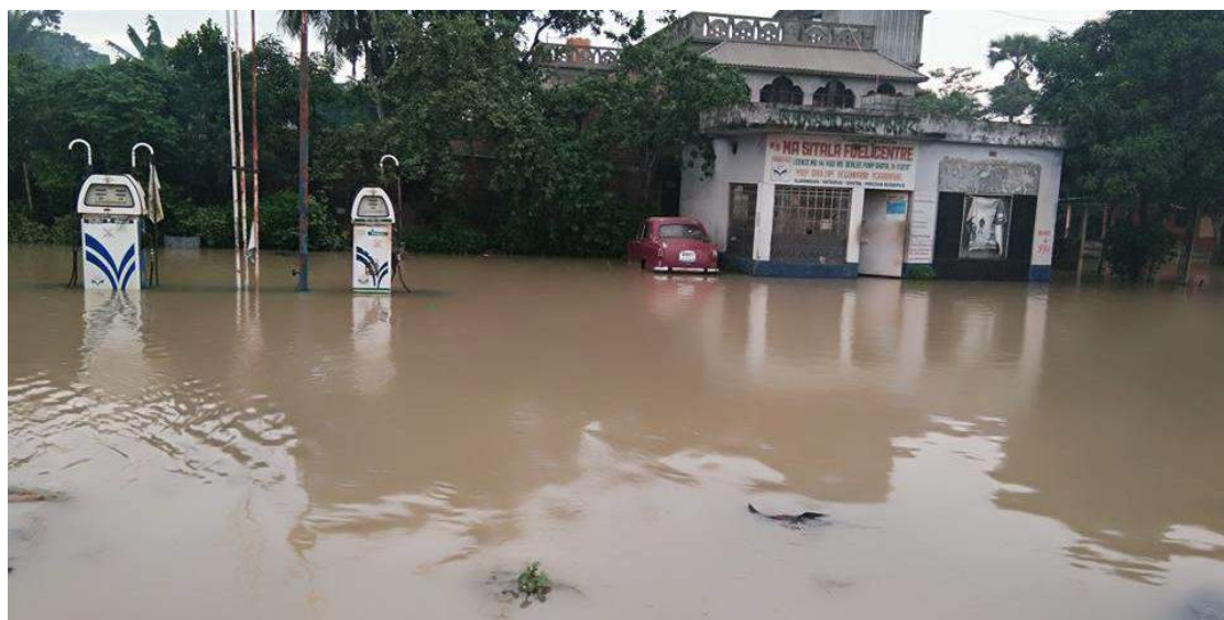
Petrol Pump under Flood Water at Paschim Medinipur
