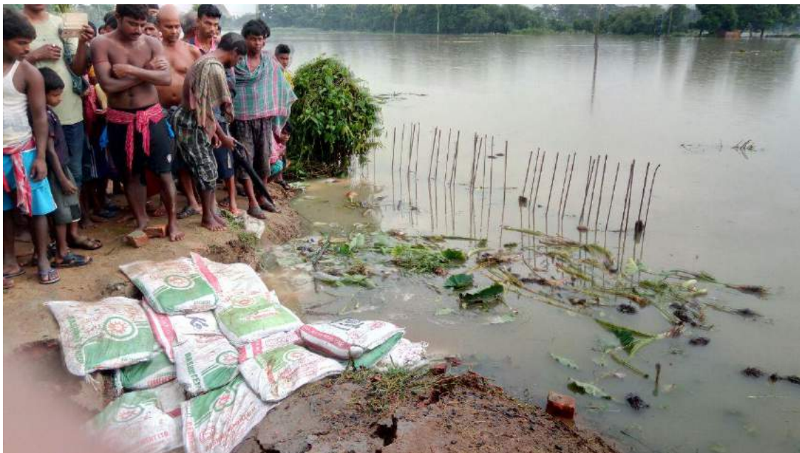
Repairing of Damaged Road at Howrah
