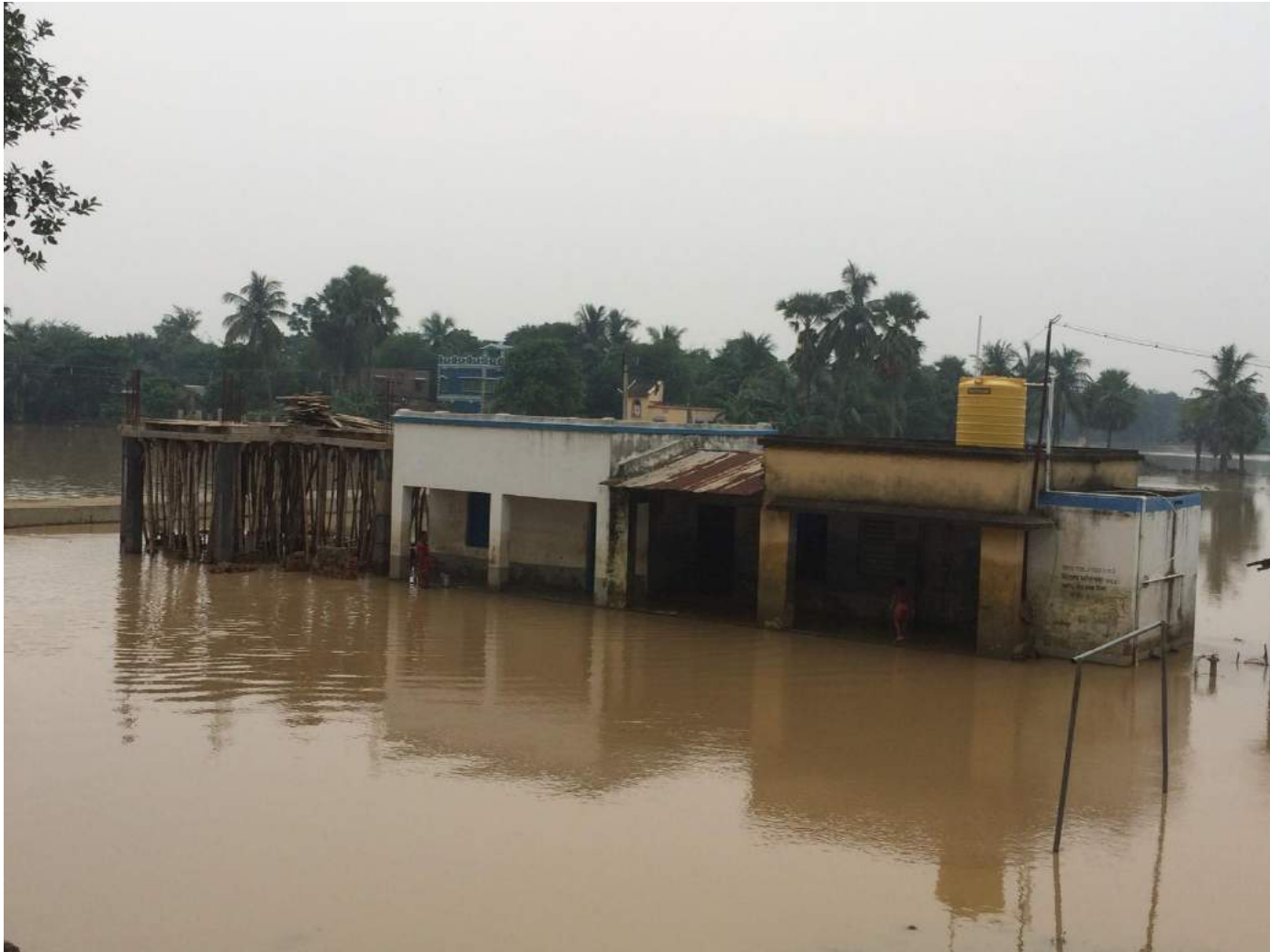
Figure10: Flooded School Building at Village - Chitkola, Jangipara Block, District – Hooghly
