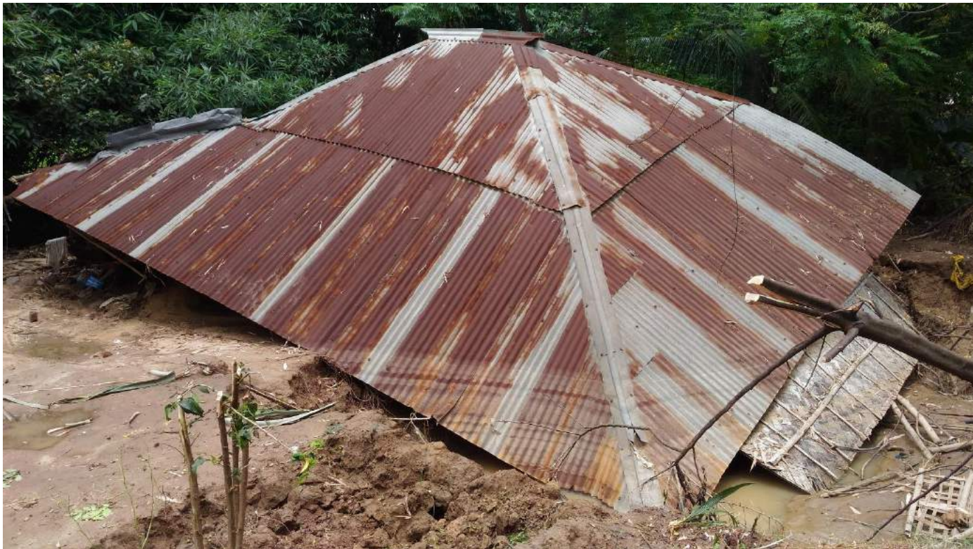
Figure 16 Fully Damaged House at UttarnityanandapurSamitimana, Radhamohanpur GP, Block - Sonamukhi, Bankura
