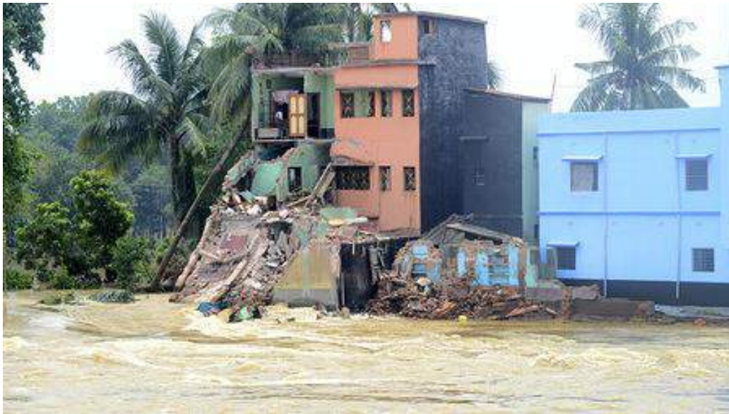
House Collapsed at Ghatal, Paschim Medinipur
